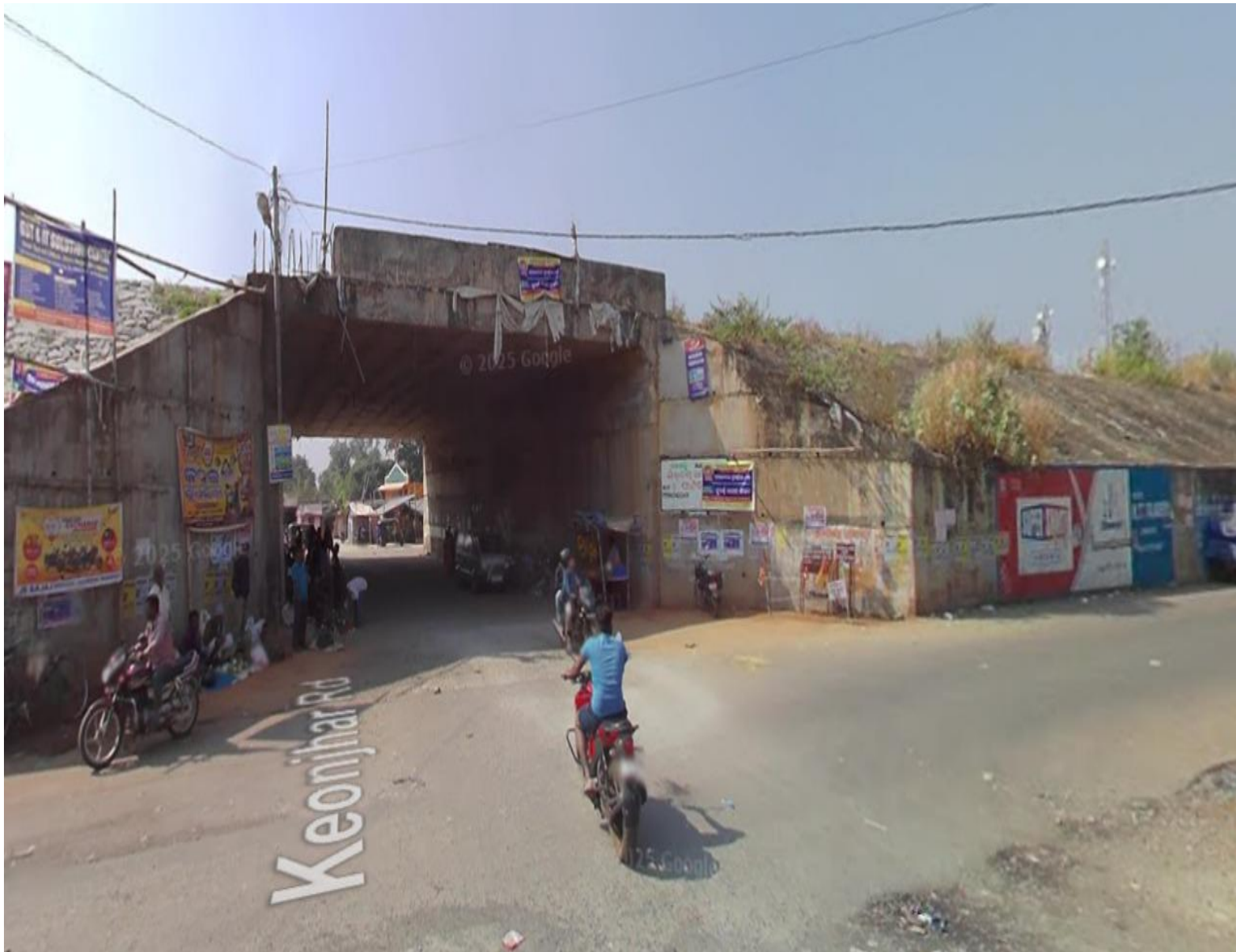
IMAGE: EXIT HIGHWAY ; RiskLevel: MEDIUM ; Coordinates: 21.4928488,85.8364455 (162 Km)
